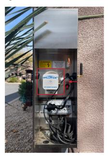
6. Thread the antenna wire onto the antenna port of the Smart Socket 3.0.
