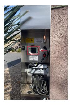
**3.** Feed the antenna wire through the photocell knockout.
