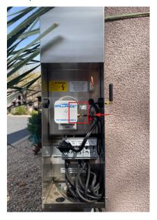
7. Plug the timing mechanism cord into the bottom of the Smart Socket 3.0.
