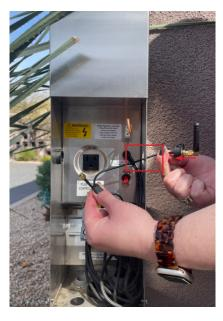
4. Press the antenna plug firmly into the photocell knockout.
